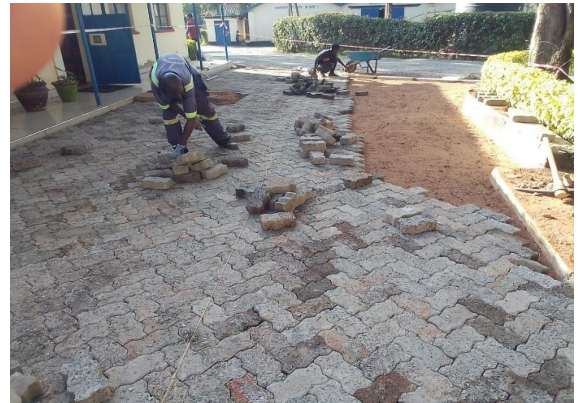
Fixing the cabro-blocks
