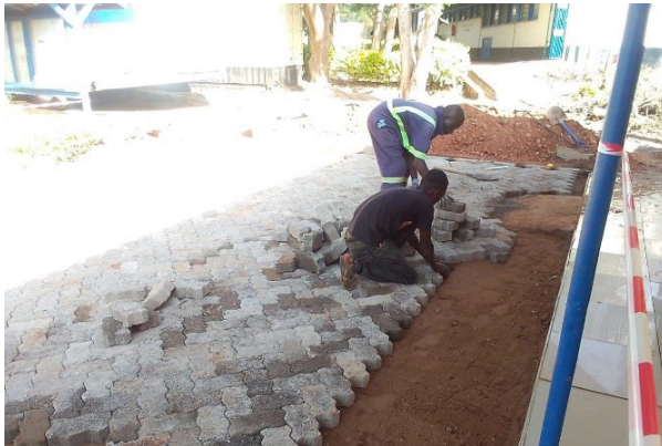
Fixing the cabro-blocks
