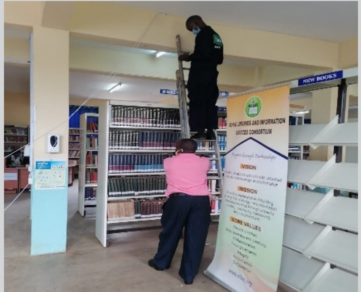
Suppliers installing intrusion control system in the library
